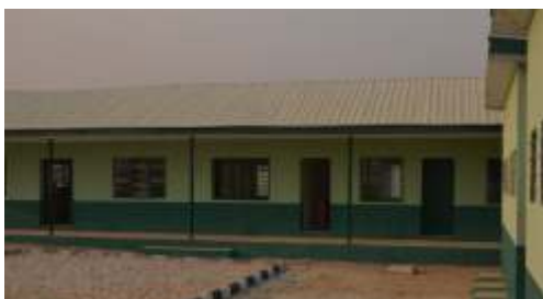
Finished Classroom Block
