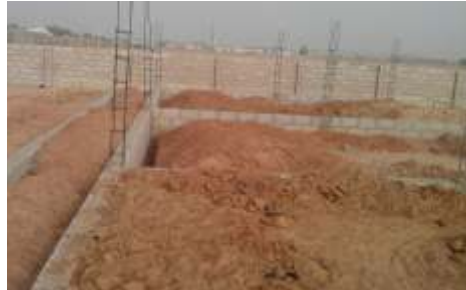
The first blocks are laid on site
